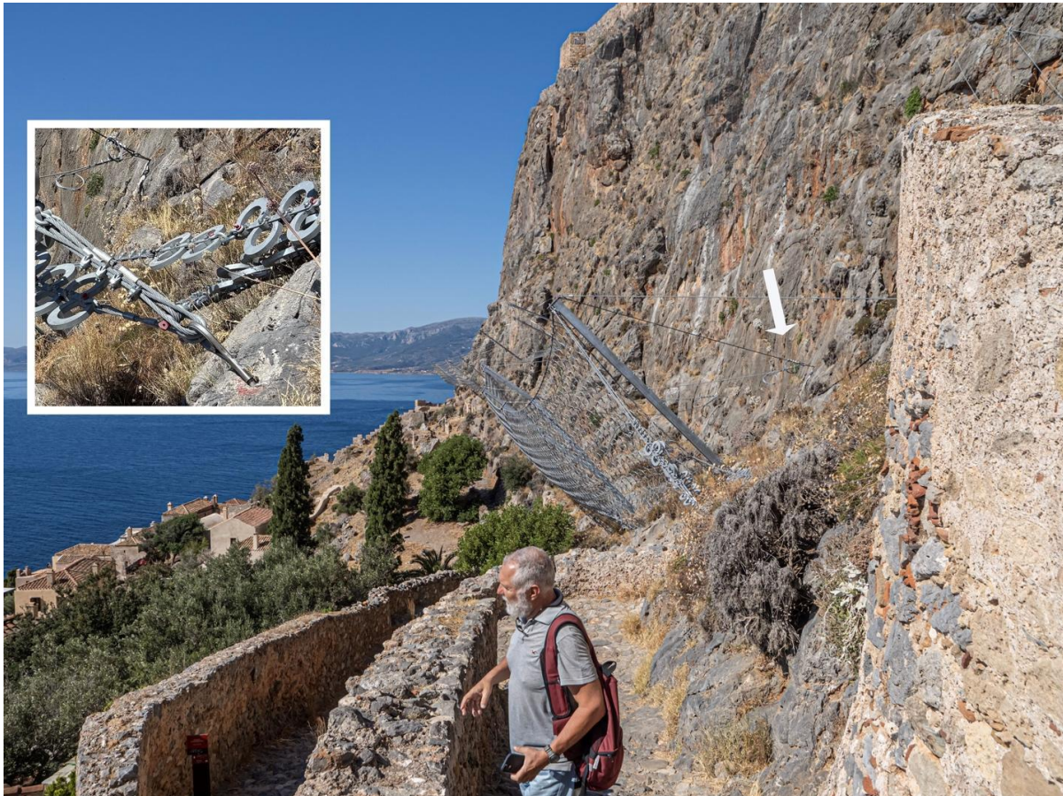
Fig. 3 Annex. The rockfall barriers, as seen from the path to the upper town, create a jarring visual impact. The invasive metal anchors and modern materials stand in stark contrast to the historic character and traditional materials of the site (Europa Nostra).
