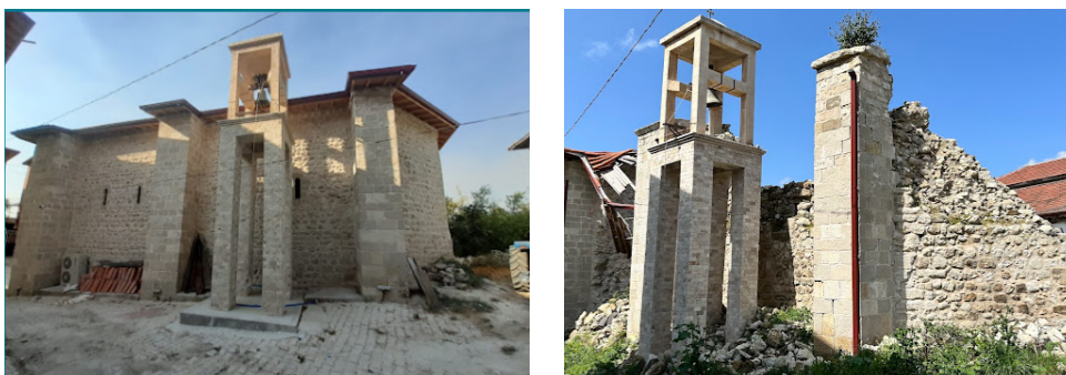
Fig. 7, 8: Tokaçlı church, before and after the earthquake (images: Google Maps)
