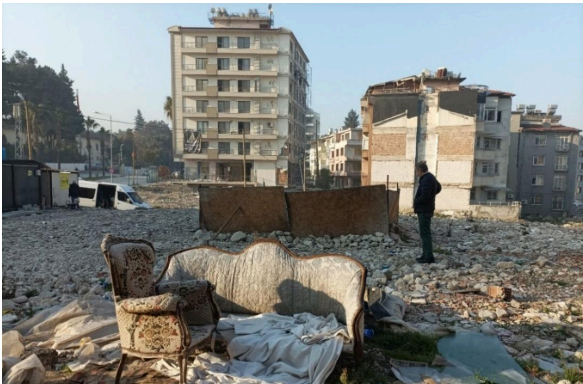
Fig. 19: Antioch. Photo shows a demolished building after the earthquake damage. On the back, buildings are damaged but still standing.
