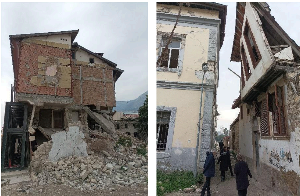
Fig. 5,6: Damaged buildings from the 2023 earthquake in Antioch city center
