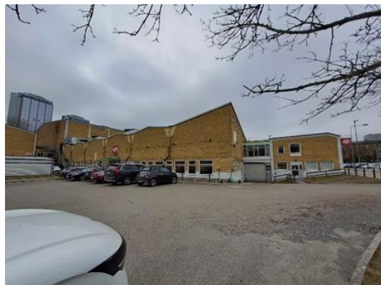
Boiler house beside main swimming hall building
