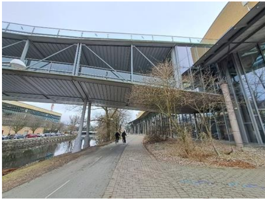
Foot + cycle paths pass under passageway to carpark
