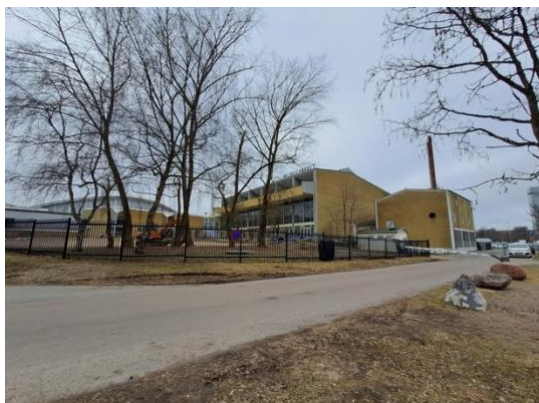
50m indoor pool behind trees. Right: Boiler house
